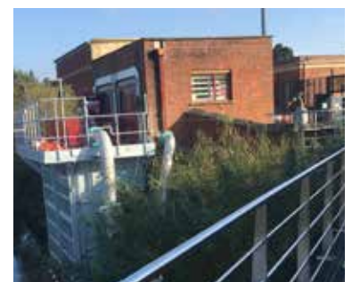
The eel screen support structure at MWTW 1941 intake
