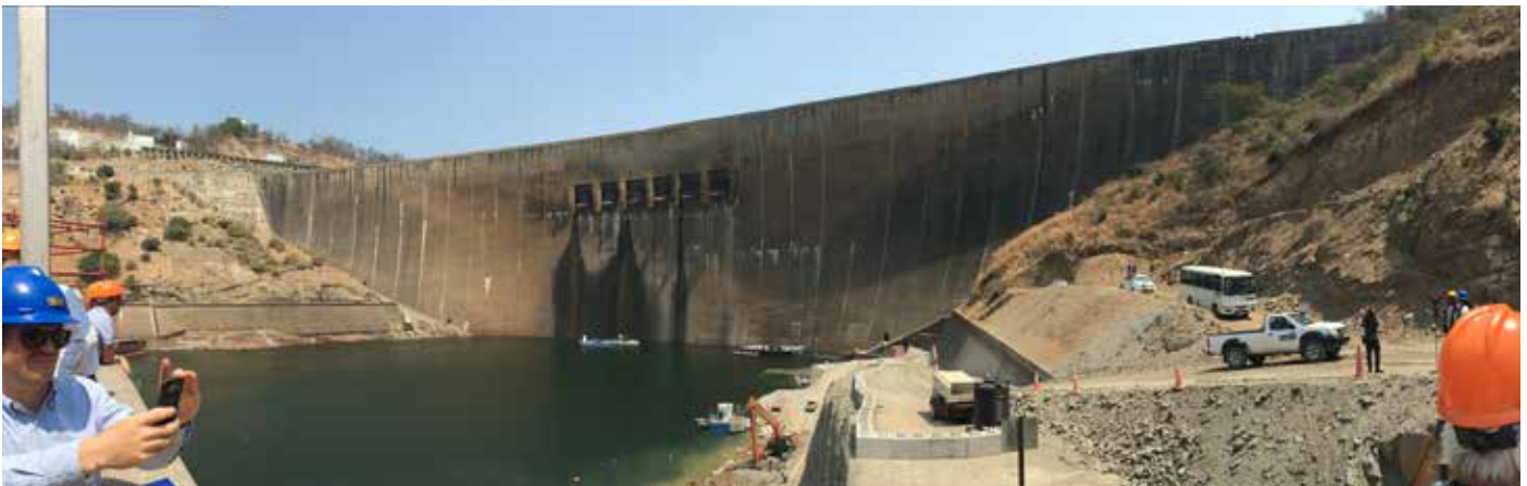
Kariba Dam rehabilitation
