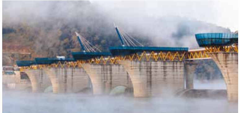
Nakdong weir with five rising sector gates
