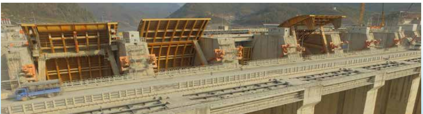
Xayaburi HEP Spillway
