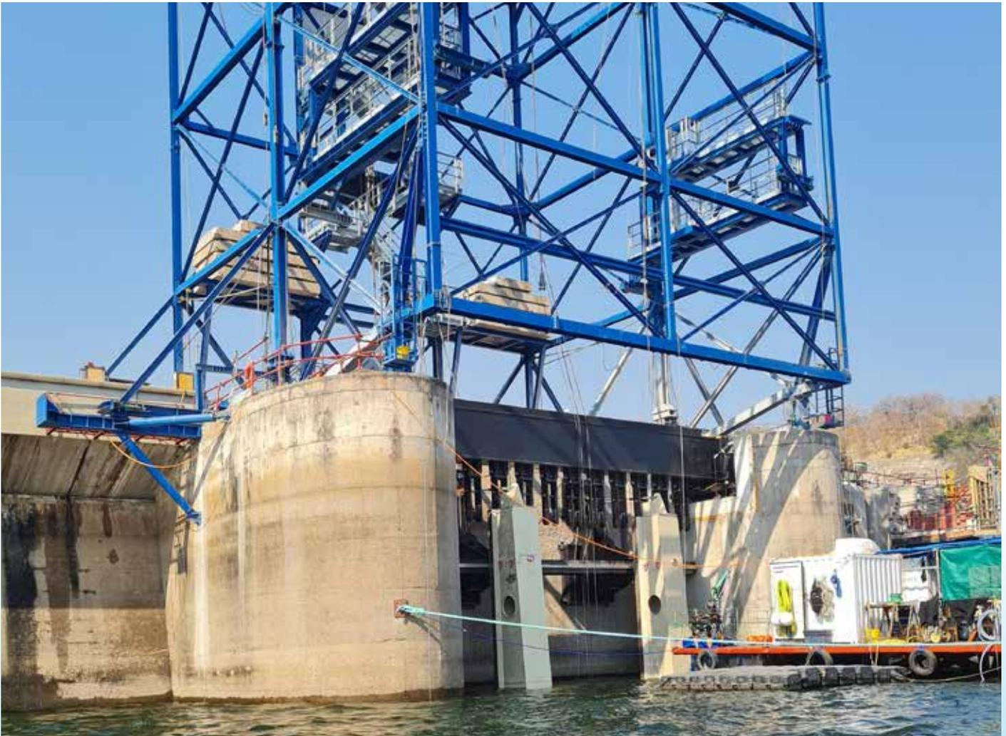
Portal frame used to lift and handle the needles
