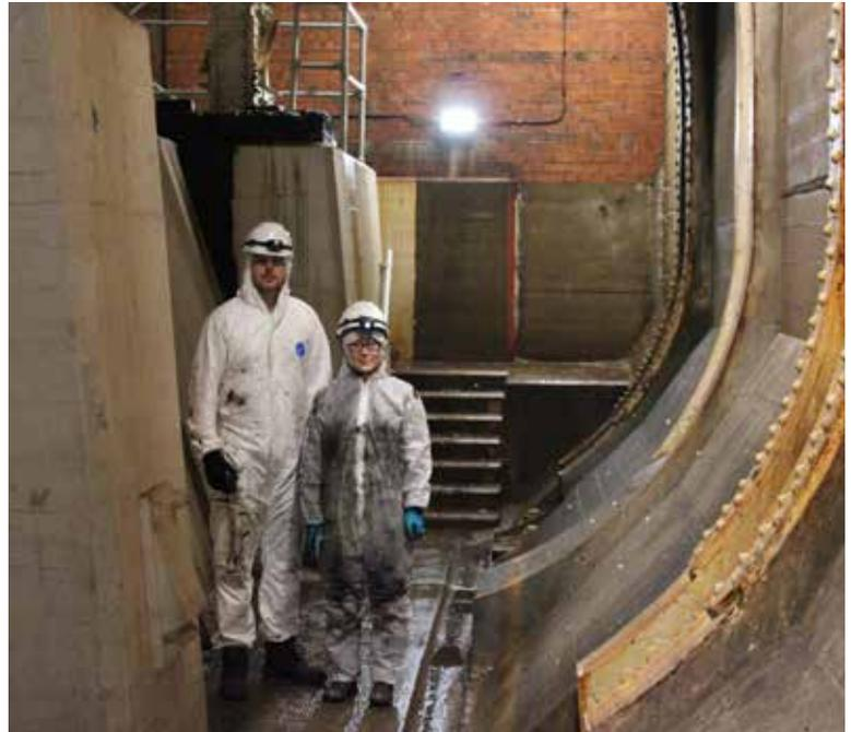
The long and the short of it; KGAL Technician Billy Owen and Engineer Yue He inside the bascule chamber. During lifting, the heel of the deck comes down into where they are standing.
