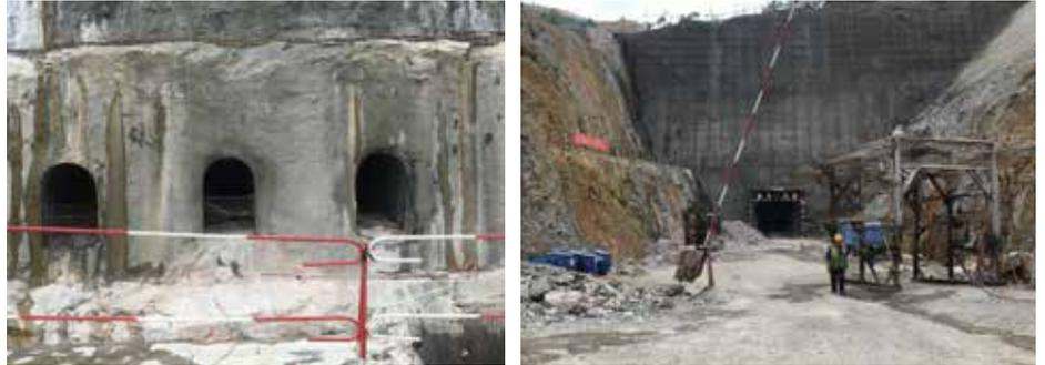
The intake tunnel and high-pressure outlets to the power house under construction at NK3
