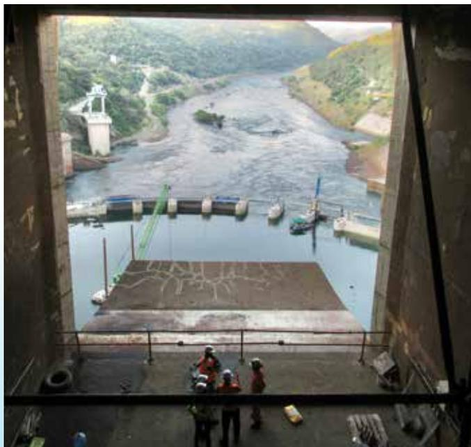
Sluice 6 was the first to be dewatered using the KGAL designed cofferdam. Before the scaffolding was installed, there was a brief opportunity to fly a drone up the 35m height of the cofferdam and to the top of the portal frame used for installation of the cofferdam, as shown here:
