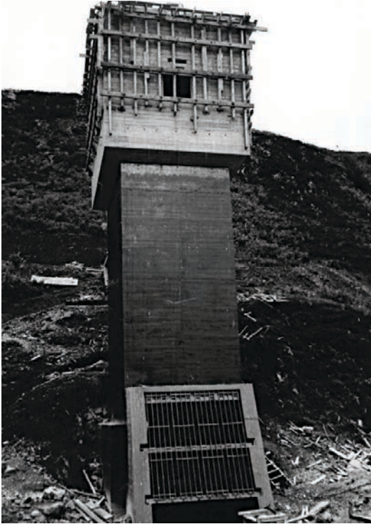
Original Intake Tower under construction
