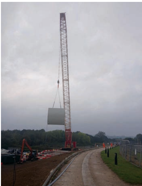
Installation of the south radial gate at LEHES
