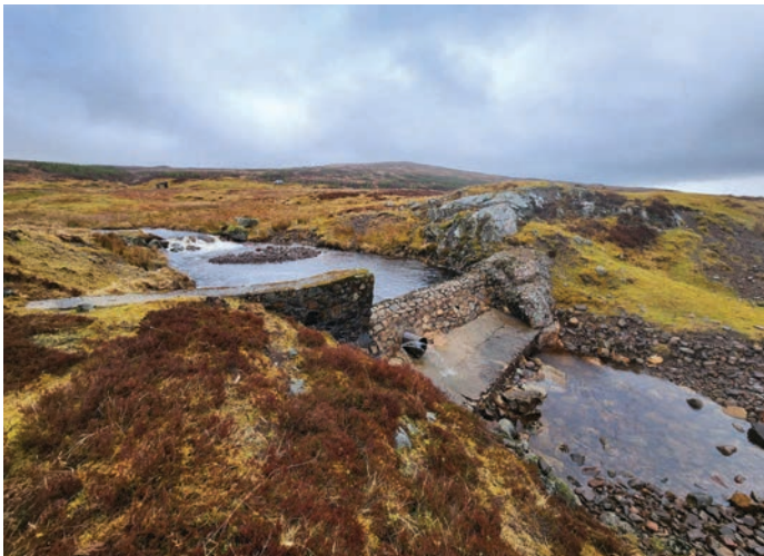
Aulich Intake diverts water to Rannoch Power Station, before it passes through Tummel, Clunie and Pitlochry Power Stations en route to the River Tay.
