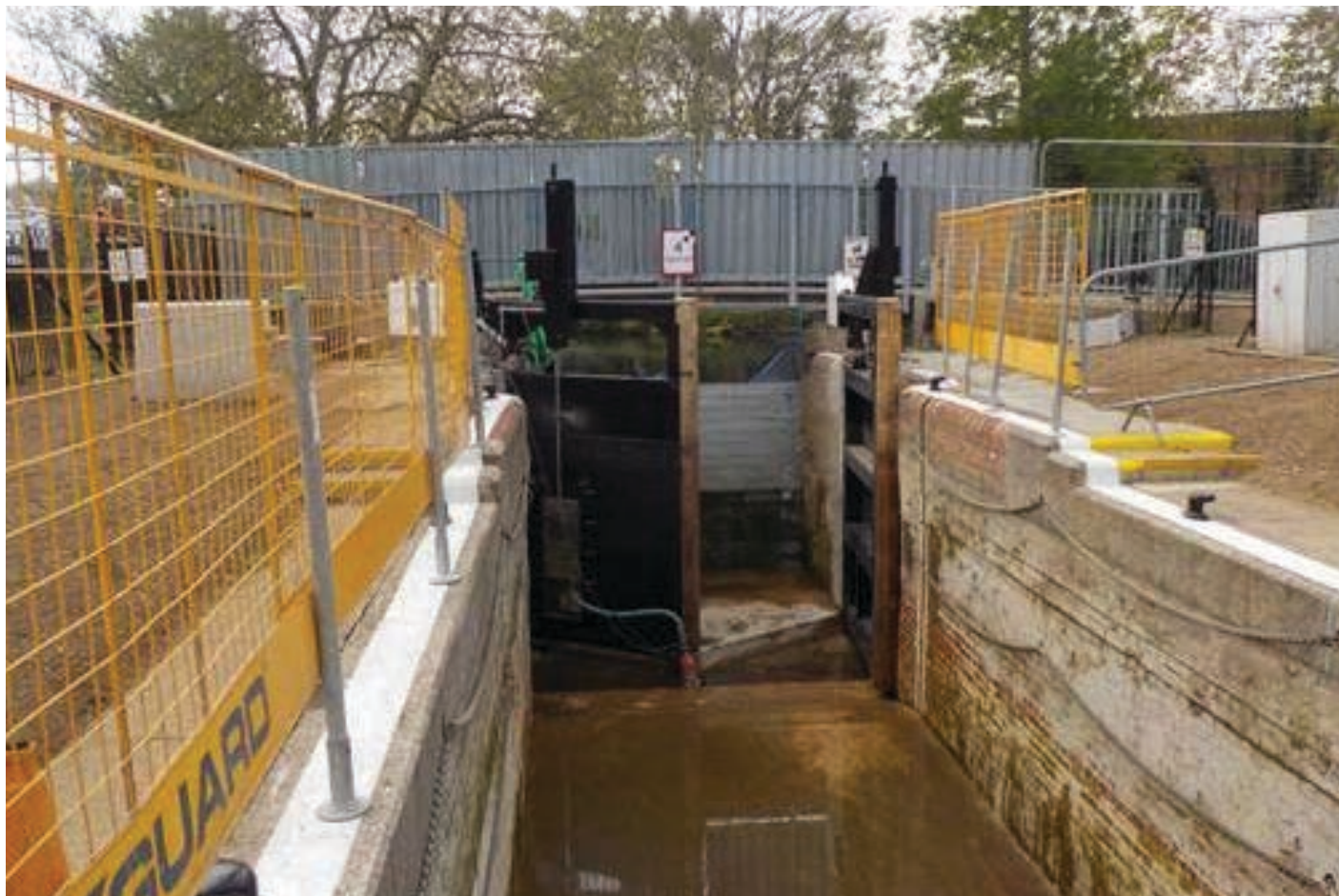
View looking downstream at the newly installed Mitre gate and associated parts in the dewatered Lock. KGAL designed stoplogs downstream of the gate
