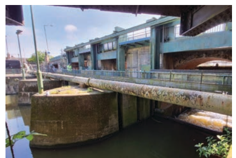
View from upstream looking downstream at sluice gates
