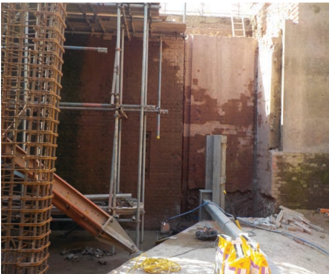
View looking along sill at new lower quoin section
