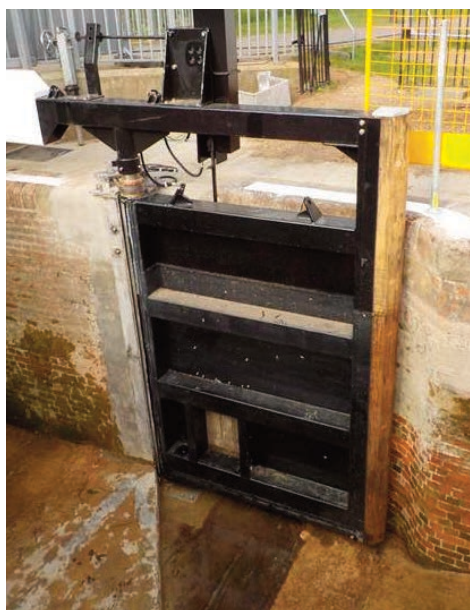
View of the right-hand side Mitre gate leaf in the open position in a dewatered lock, showing the new Sill, Quoin and Top Anchor assemblies.
