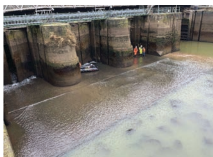
View of the pointing doors
