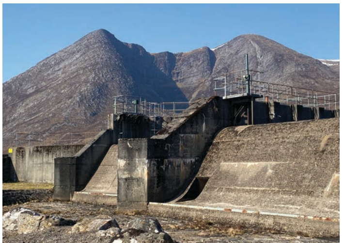
Chronin Idir Intake feeds water to Loch Fannich, the upper reservoir for Grudie Bridge Power Station, before it continues through Luichart and Tor Achilty Power Stations to the River Conon
