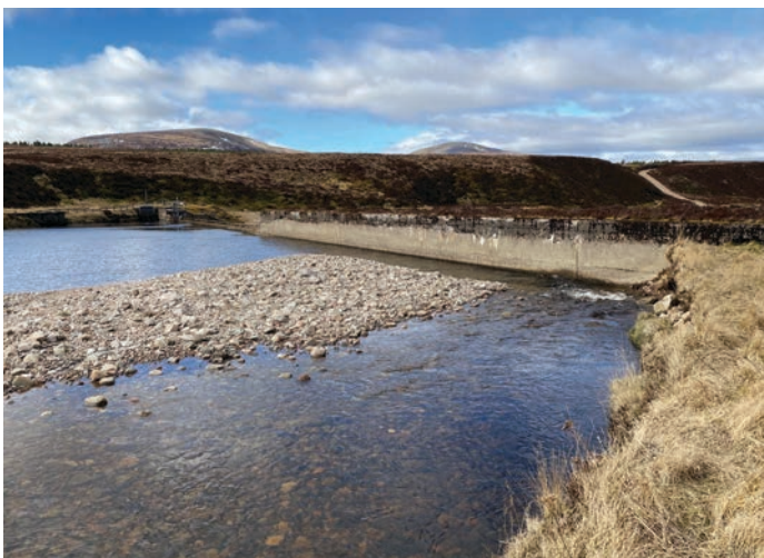
Allt Bhran Intake feeds water to Loch Erich via Loch an t-Seilich, Loch Cuaich and Cuaich Power Station, before it continues through the Rannoch, Tummel, Clunie and Pitlochry hydropower cascade to the River Tay.
