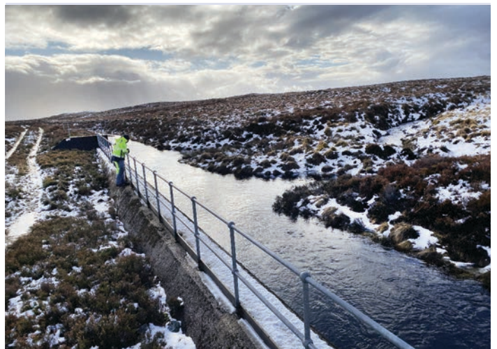
Chuil Intake is one of three intakes feeding an aqueduct to Loch Shin and Shin Power Station, located within the Flow Country World Heritage Site in Sutherland.
