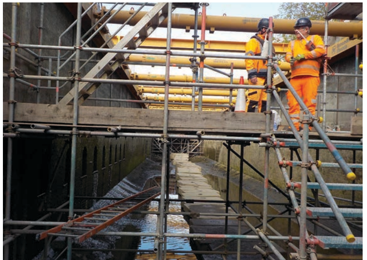
View looking downstream in dewatered lock
